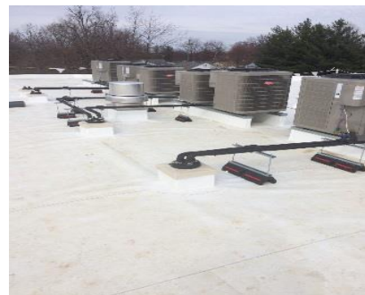
Pictured Left is the trench drain installation in the apparatus bay and picture Right is the roof mounted AC units with refrigeration piping.
