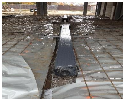
Pictured Left is the trench drain installation in the apparatus bay and picture Right is the roof mounted AC units with refrigeration piping.
